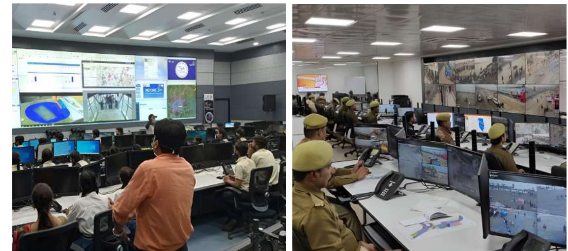
Integrated Command and Control Centres in smart cities of Indore (on left) and Prayagraj (on right)
