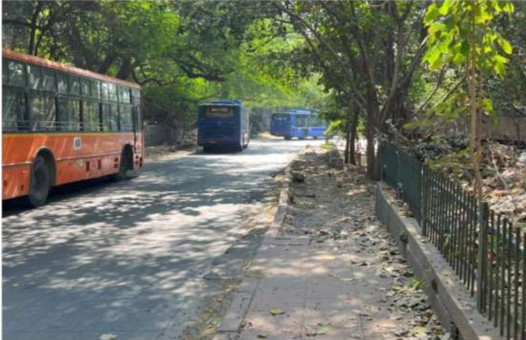
Broken and discontinuous footpath
