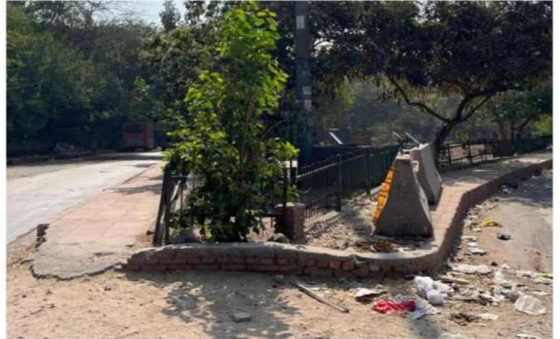
Footpath obstructed by garbage and cement barricades
