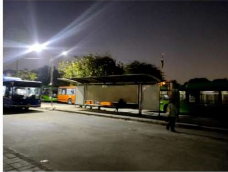
No functional lights at the waiting area, leading to dark spots
