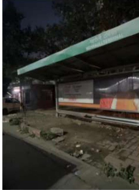
Absence of lighting at the waiting area
