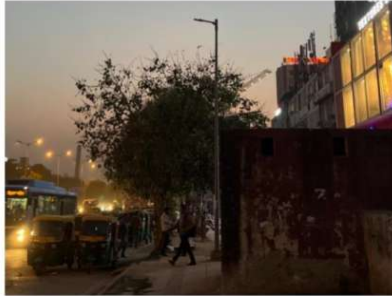
Inconsistent illumination due to non-functional streetlights on the footpath
