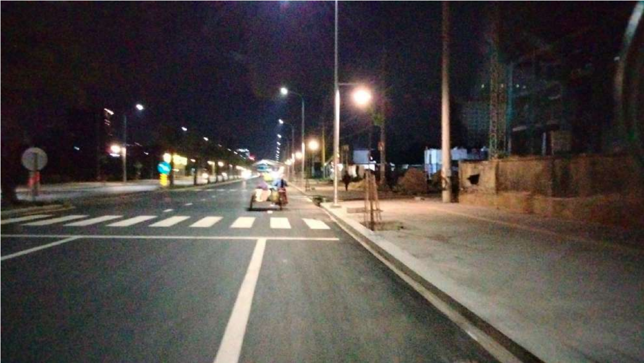
Image 11: Proper pavement in 2021
