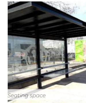
Bus stop shelter
