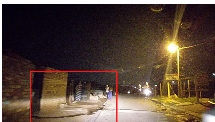
Image 10. Street with broken patch
