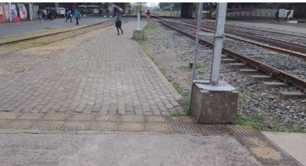
Image showing discontinuous tactile paving on the platform at Dematogoda station
