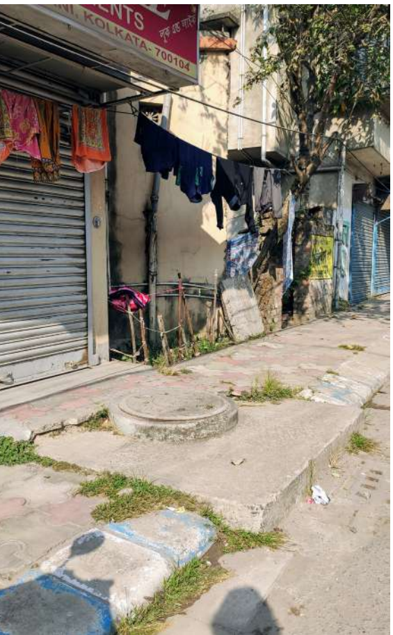
Image 17: Manhole jutting out
