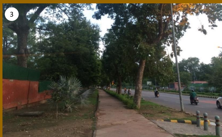
Motilal Nehru Marg. The road has a footpath and a ramped egress. But the bollards at the edge prohibit movement of wheelchair. While the bollards are necessary to prevent entry of vehicles, they should be placed so as to allow smooth movement of pedestrians and people on wheelchair. Also tactile paving needs to be incorporated along the entire length of the footpath including the ramps.
