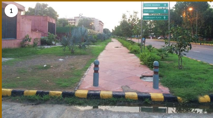
Motilal Nehru Marg towards Akhbar Road. The footpath should have a ramped interface with the road.
