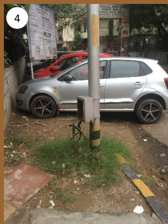
3 4 Seen here in pics3 and 4 are the edge conditions of the footpath with the road. The ramp needs to be built at a slope of 1:15 to ensure comfortable movement of people on wheelchair and women with prams. The footpath needs to have a kerb height of 150mm such that vehicles cannot be parked on it.
