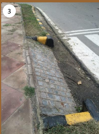
3 4 Seen here in pics3 and 4 are the edge conditions of the footpath with the road. The ramp needs to be built at a slope of 1:15 to ensure comfortable movement of people on wheelchair and women with prams. The footpath needs to have a kerb height of 150mm such that vehicles cannot be parked on it.
