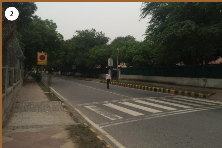
2 Data Ram Bhutani Marg. As seen here in pic2, there is a ramped ingress/egress along the zebra crossing. However, the two ramps should be exactly aligned with the crossing. Currently, this is only on one side of the road and on the other side the zebra crossing meets the kerb stone.
